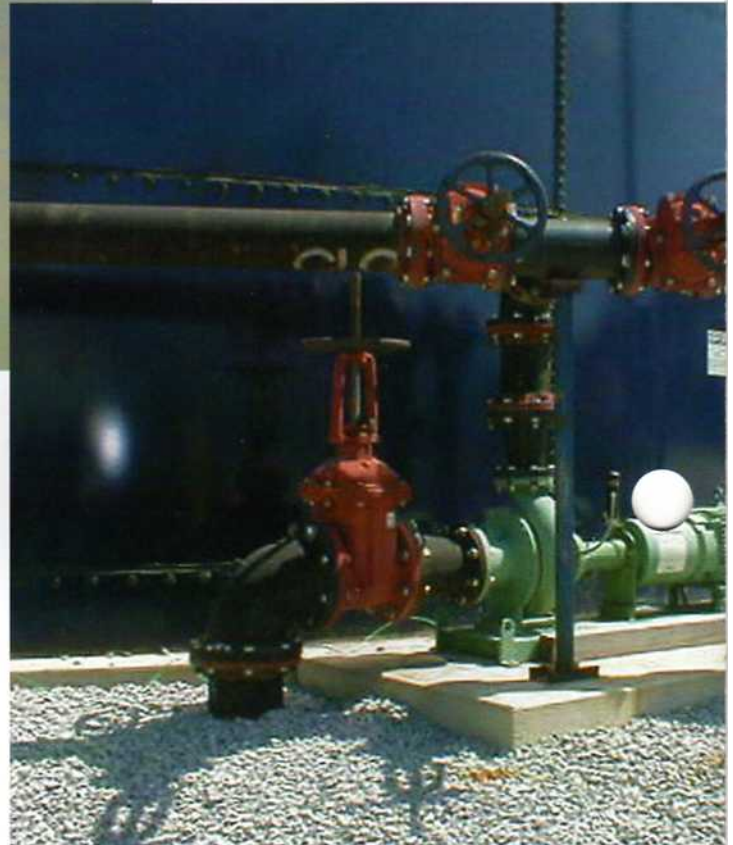
Powerful floor-mounted nozzles efficiently mix very large volumes of liquid while chopper pumps reduce solids.
